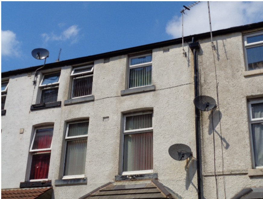
Insensitively positioned satellite dishes in Foxhall Conservation Area
