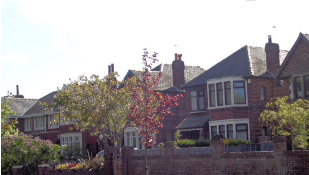
Chimneys in Stanley Park Conservation Area
