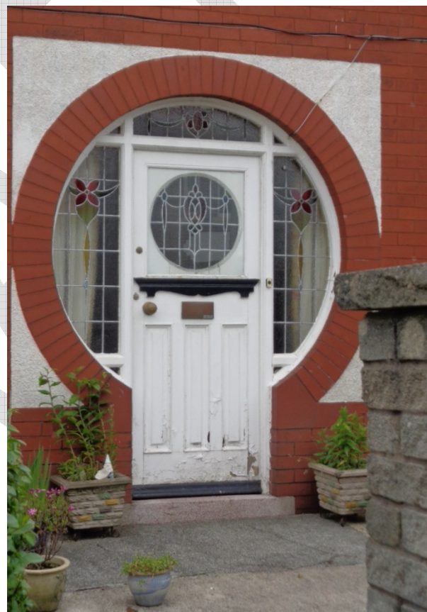
Original 1930s front door with leaded and stained glass
