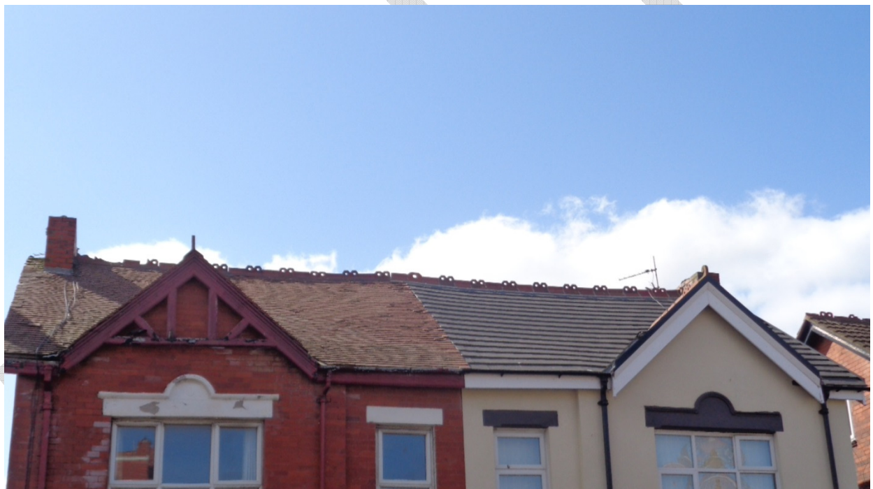
Red clay tile roof covering to the left and modern roof tile to the right of this pair of semi-detached villas
